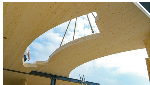
FIGURE 15 Modular Mass Timber Construction
