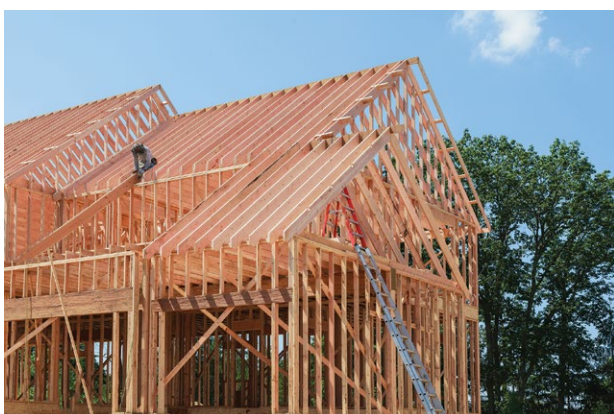
FIGURE 5 On-site Construction Typical of the United States of America and Canada
