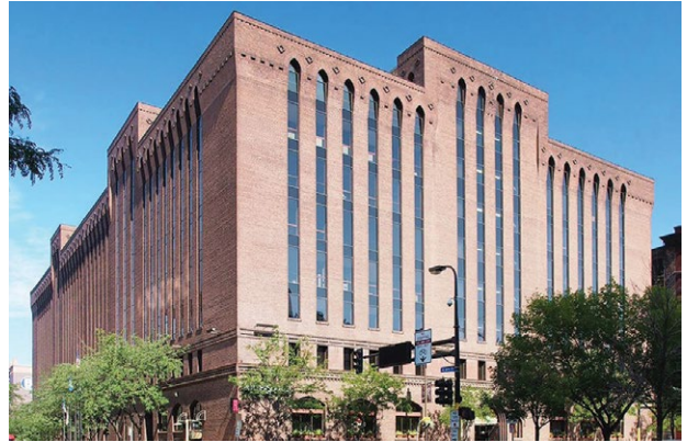
FIGURE 11 Butler building, Minneapolis, United States of America
