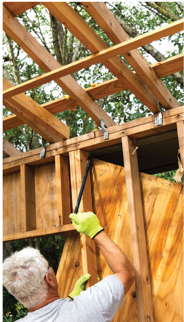
FIGURE 19 Deconstruction for Building Materials Recovery
