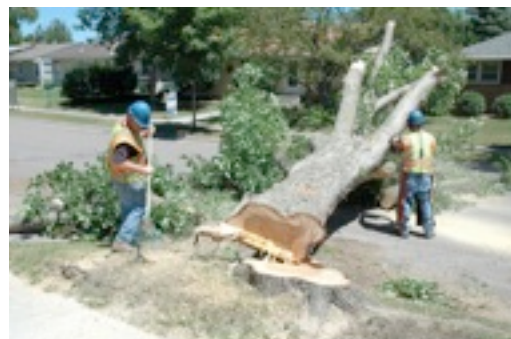
Figure 3. Tree removal in Minneapolis.
