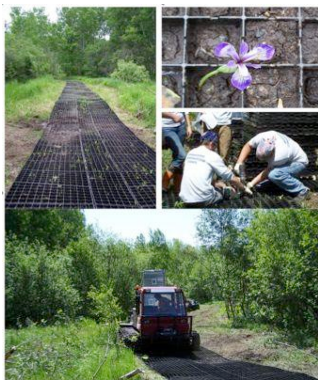
Use of geoblock to reduce trail construction impacts.
