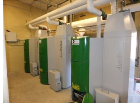
Figure 6. Interconnected Modular Design
