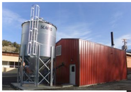
Figure 5. Pellet Silo and Boiler Housing Building
