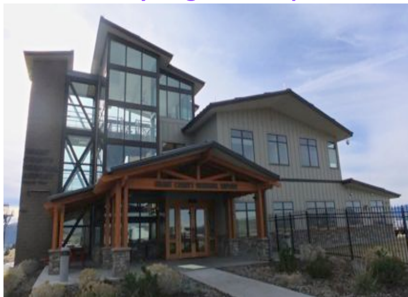
Figure 10. Grant County Regional Airport Airbase Building
