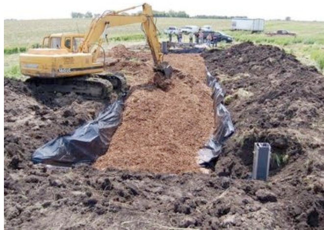
Figure 5. Installing a Denitrifying Woodchip Bioreactor
